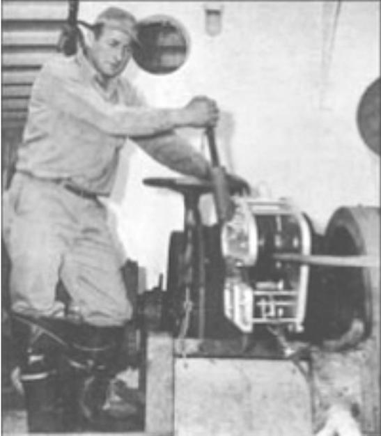
When trawling, a pair of 750-N Meters enables the winch men to accurately synchronize their winches and make corrective changes of warp settings. Meters avoid errors caused by warps stretching in service. This is particularly important during mid-water trawling. Avoid costly trips to port for remarking damaged cables.
